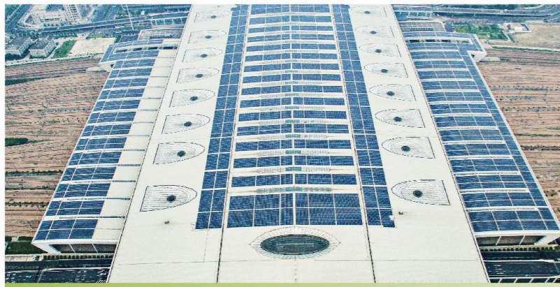
Hangzhou East Railway Station project capacity 10MW
